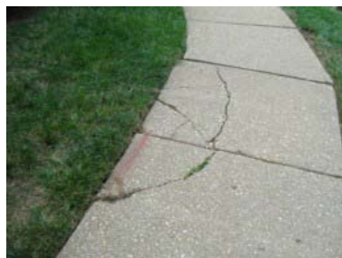
Typical Cracked Sections of Sidewalk
