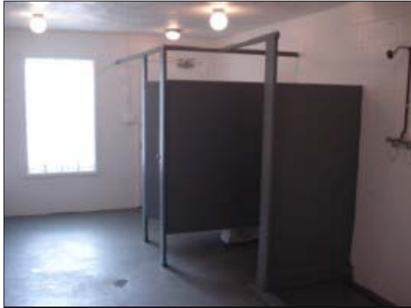
Photo #7. Bath House Toilet Room
