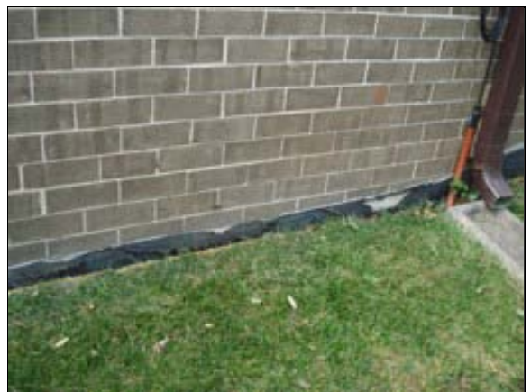
Photo #6. Foundation Sealing
