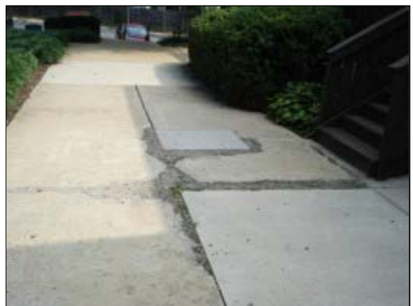
Photo #12. Courtyard Concrete
