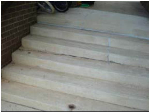
Photo #3 Concrete Stairs
