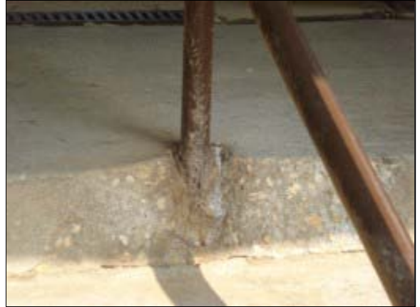
Photo #2 Hand Rail at Concrete Stair
