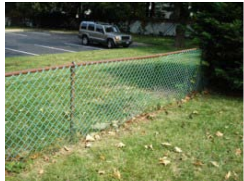
Chain Link Fence
